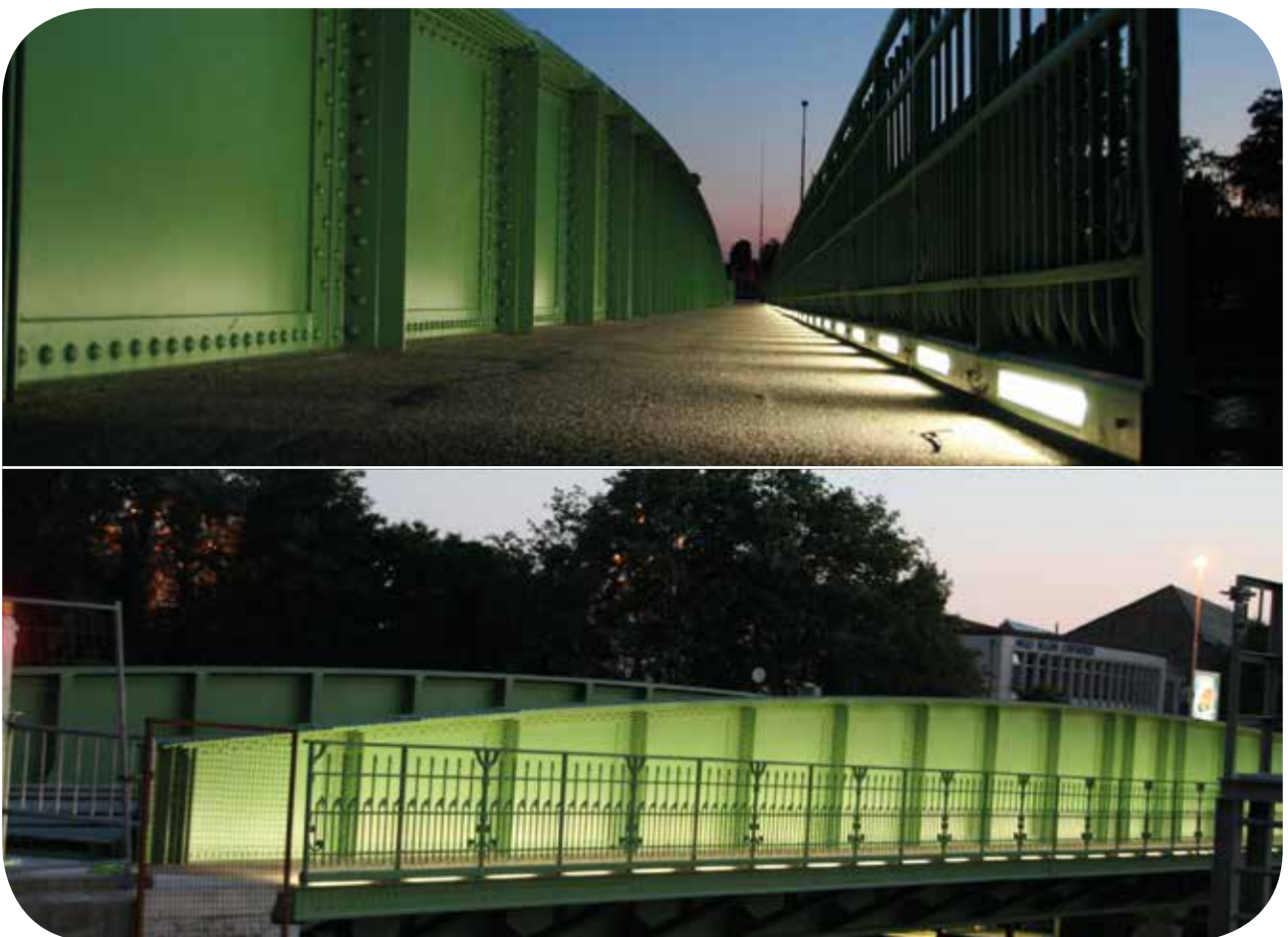
Railroad bridge Wiedauwkaai with LED lighting
